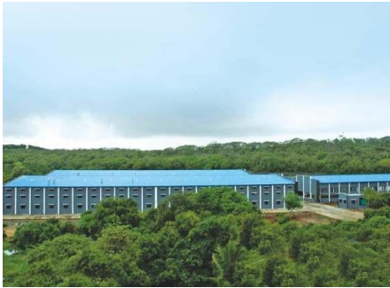
DG Set Manufacturing Unit-Kalsar, Gujarat
