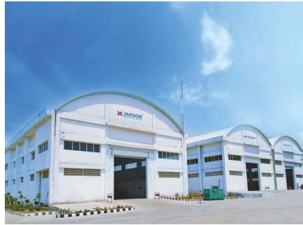
DG Set Manufacturing Unit 1-Kathua, J&K
